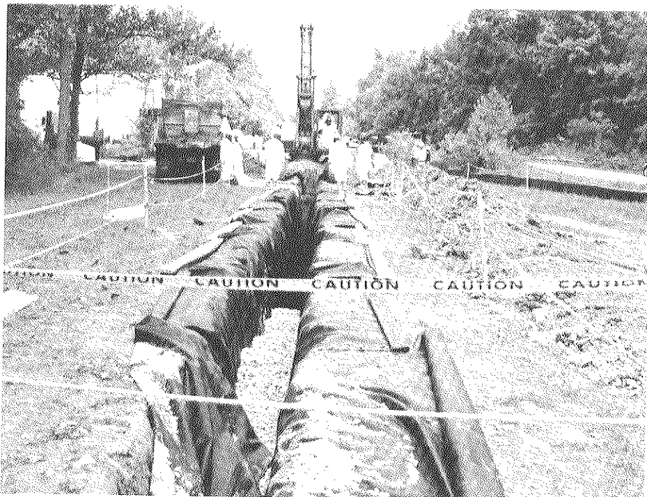
Workers have completed a trench system to capture contaminated ground water that might otherwise have reached Little Beaver Creek. The 655-foot long, nine-foot deep trench collects water for treatment before it is discharged to the sewage treatment plant.
